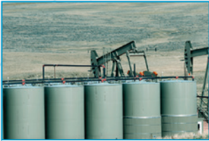
Bulk Fuel Storage and Distribution
